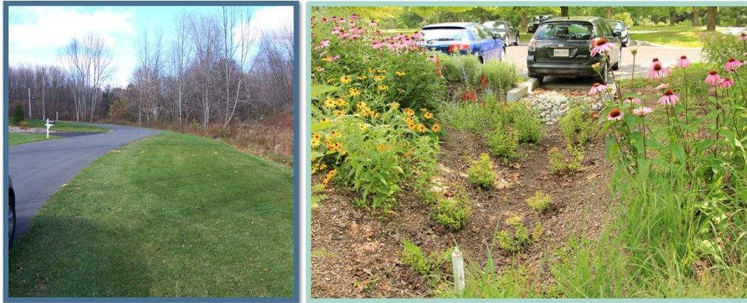
Figure 4: Grass Filter Strip and Bioretention
