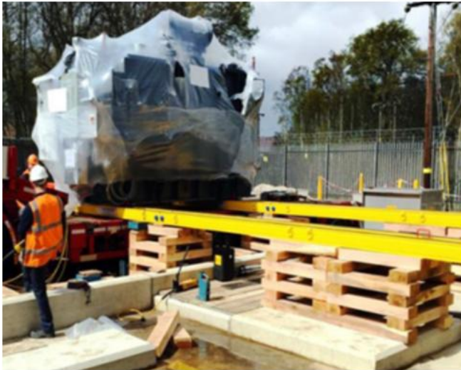
(a): Jacking system supporting large vehicle
