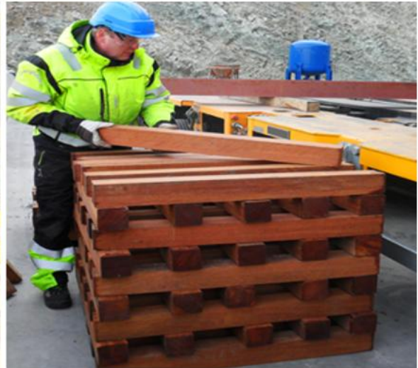
(b): Stacked Jacking beams
