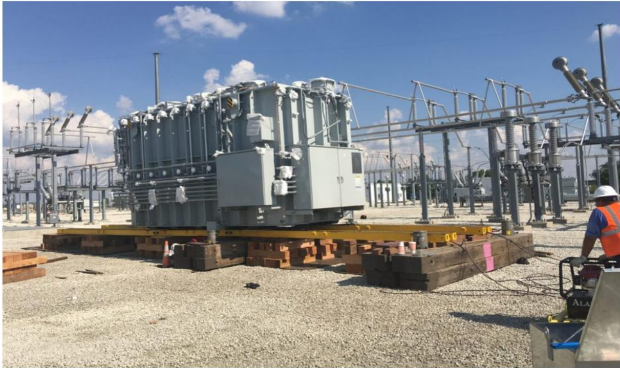
Figure 2.15: Tropical hardwoods in low-profile skidding systems
