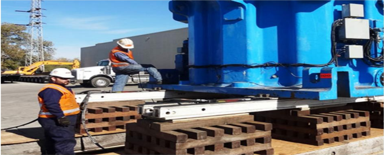
Figure 2.13: Jacking operations with Ekki beams by Hydra-Slide Ltd.
