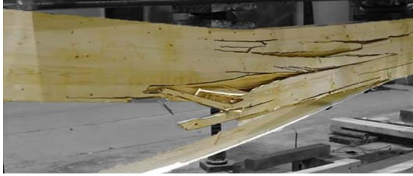
(a) Debonding of reinforcement
