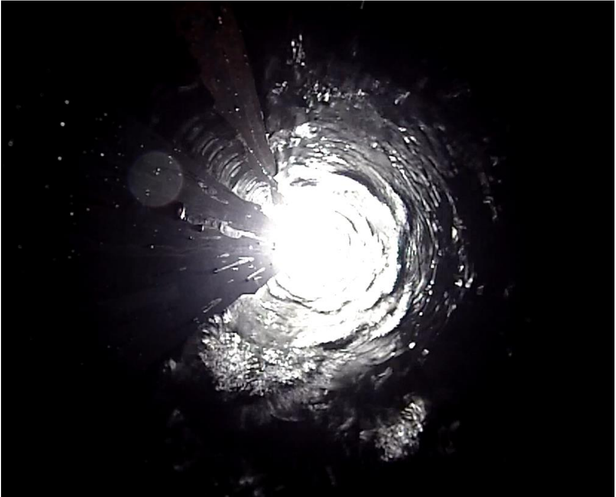
Figure 3-29: Partial falling film; the root cause behind underperformance identified in Figure 3-28.
