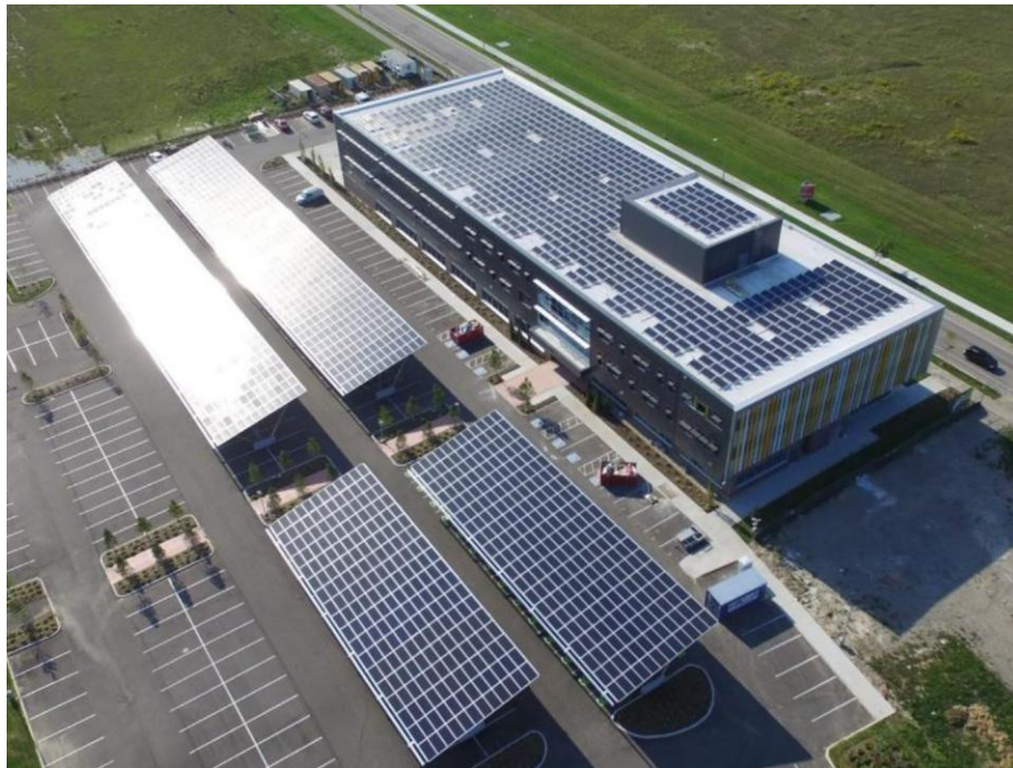
Figure 4-1- Carbon neutral office case study, located in southwest Ontario, Canada. [131]
