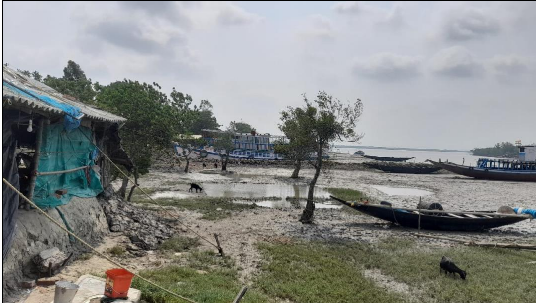
Figure 16. House Impacted by High Tidal Waters in Kumirmari, Sundarbans.
