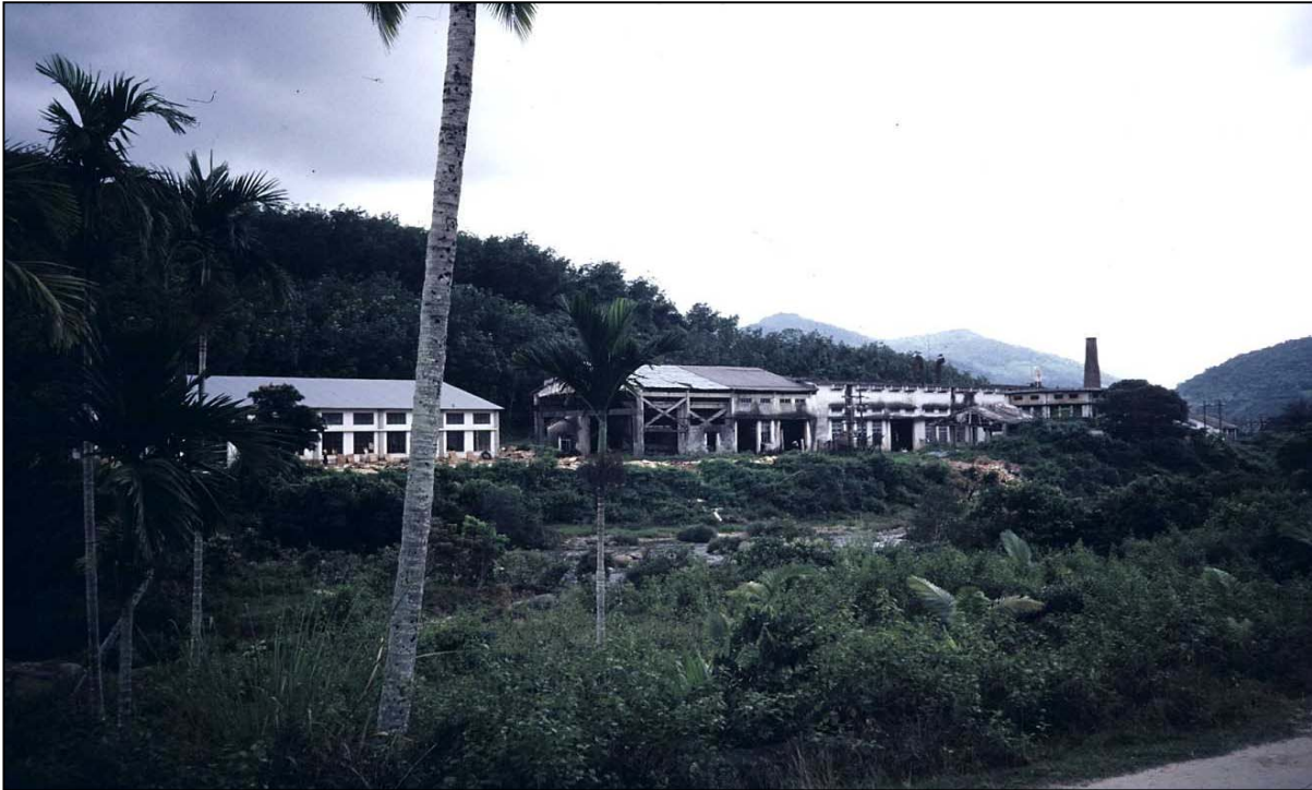
Figure 6.10: A Derelict Timber Mill, DNFP
