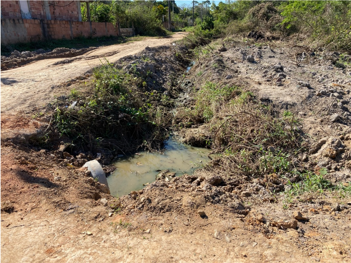
Figure 4.1. Open sewer alongside residences in Japeri-Belo Horizonte. Photo by Rodrigo Curty Pereira.
