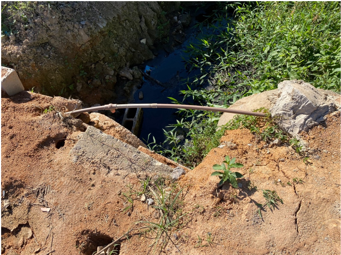
Figure 4.2. Illegal water pipe over open sewer in Japeri-Belo Horizonte. Photo by Rodrigo Curty Pereira.
