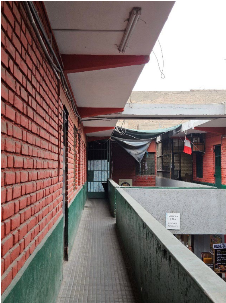
Figure 3. Picture inside of Callejón Capón. Narrow passageways lead into the second floor storage rooms and homes. Image by Author.
