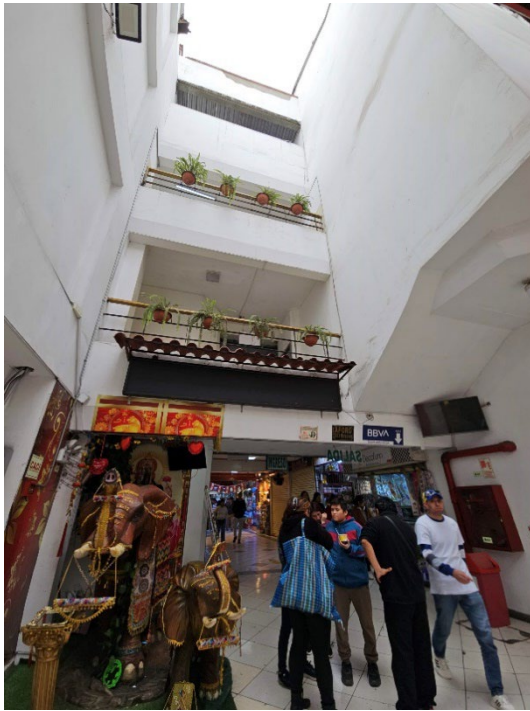
Figure 40. Interior photograph of Galeria Barrio Chino's entrance on Jirón Paruro. The entryway has no roof, allowing cool air to enter and the hot air to exhaust upwards. Image by Author.
