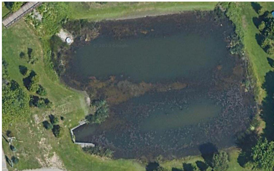
Figure 3-1. Areal view image of the stormwater pond.
