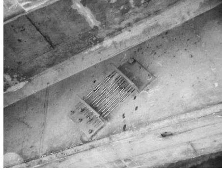
Figure 2.22. Posttensioned Fe-SMA anchored rods (Soroushian et al., 2001).
