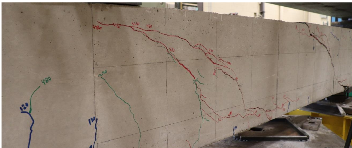
Figure A.3. Specimen N-0S: Shear Crack in Right Section
