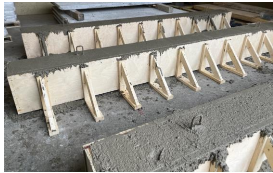
(b) RC beam cast
