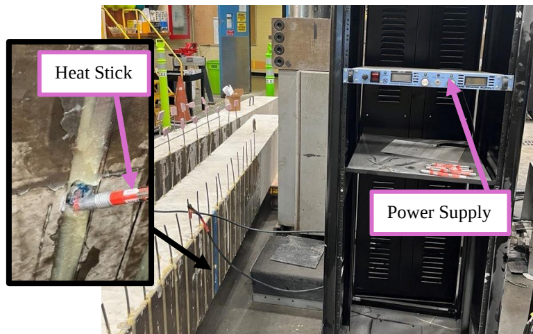
Figure 3.22. Activation of NSB Fe-SMA Strip
