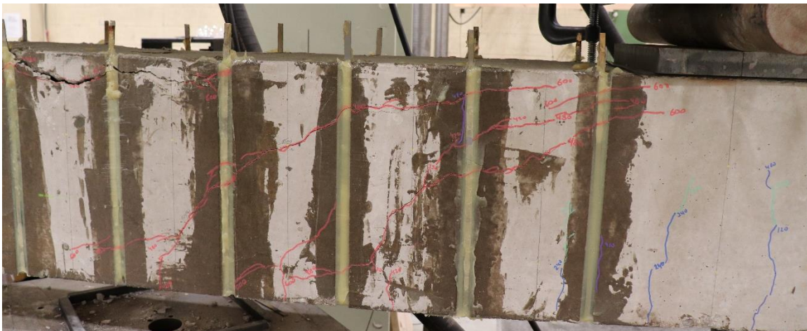
Figure A.8. Specimen A-200S-180C: Shear Crack in Right Section
