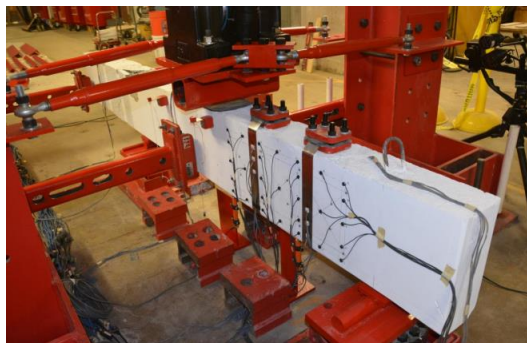
Figure 2.23. Full Wrap Fe-SMA Strengthening (Zerbe, 2020).
