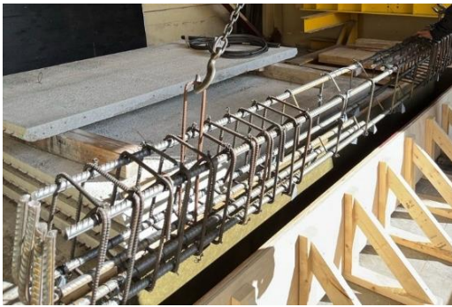
(a) Reinforcement cage
