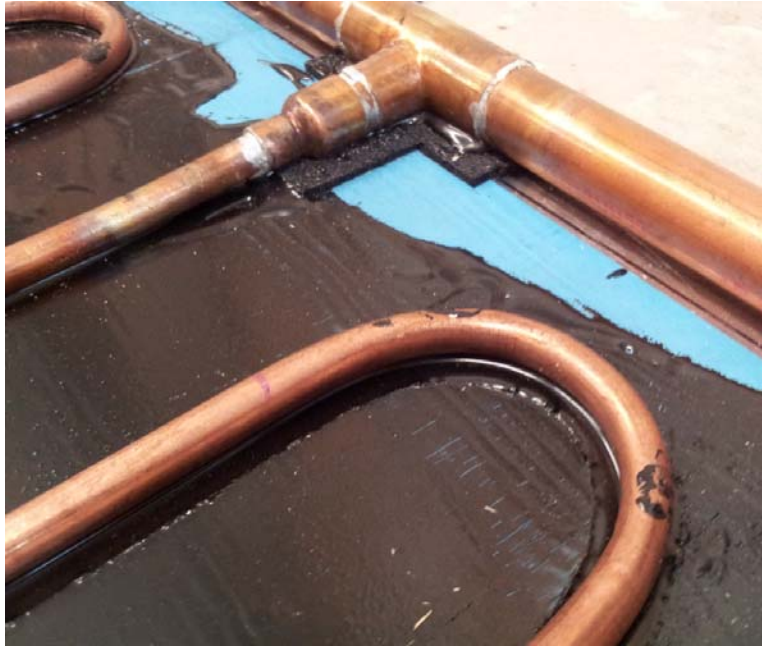
Figure 21 – Cured epoxy adhering the piping network to the aluminum plate.
