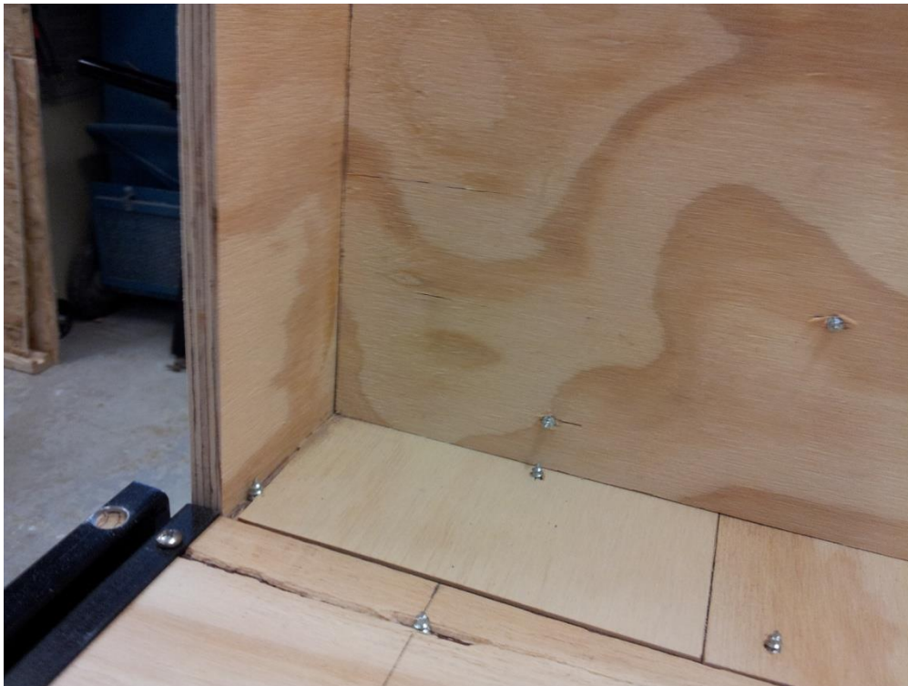
Side panel prior to edge insulation installation. Screws used to construct the side panel protrude through the plywood to help keep the insulation fixed.
