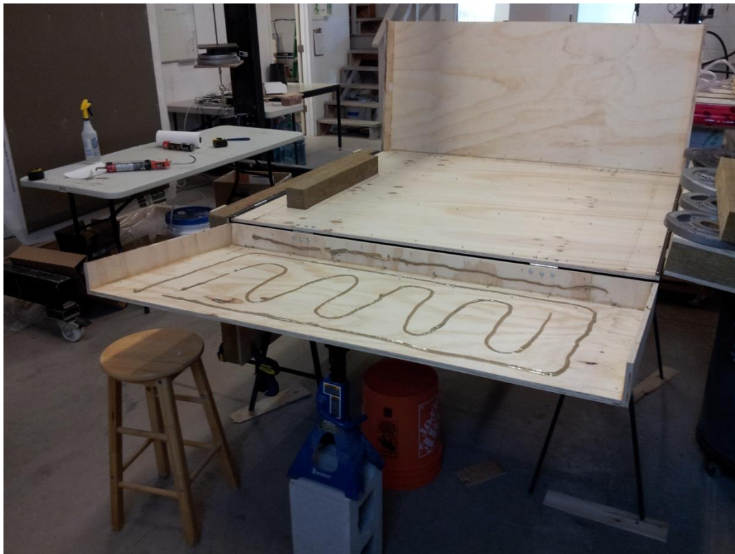
Side panels with adhesive applied just prior to edge insulation installation.
