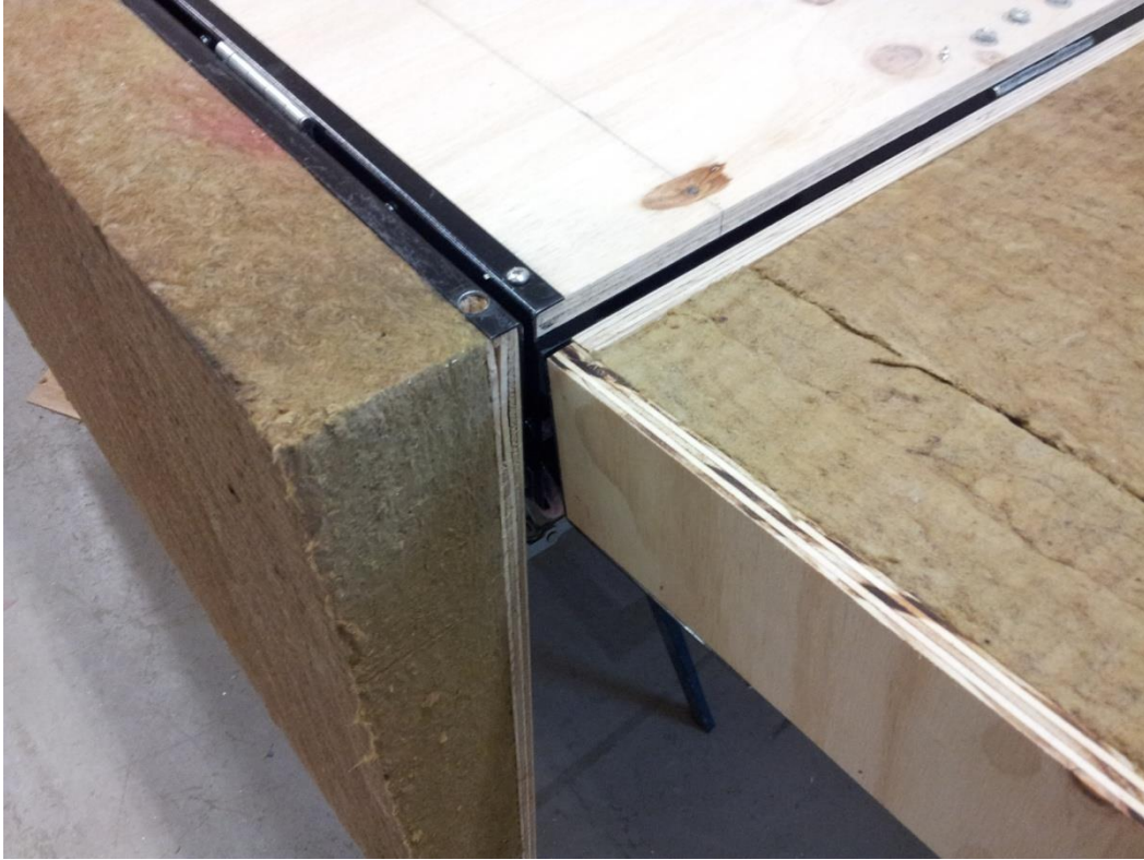
Detailed view of the edge insulation installed on the side panels.
