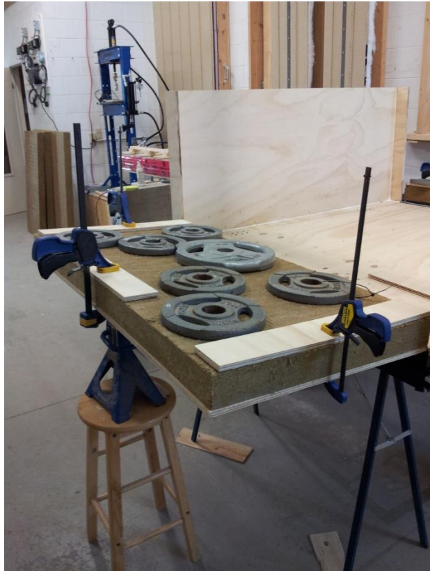
Installation of the edge insulation.
