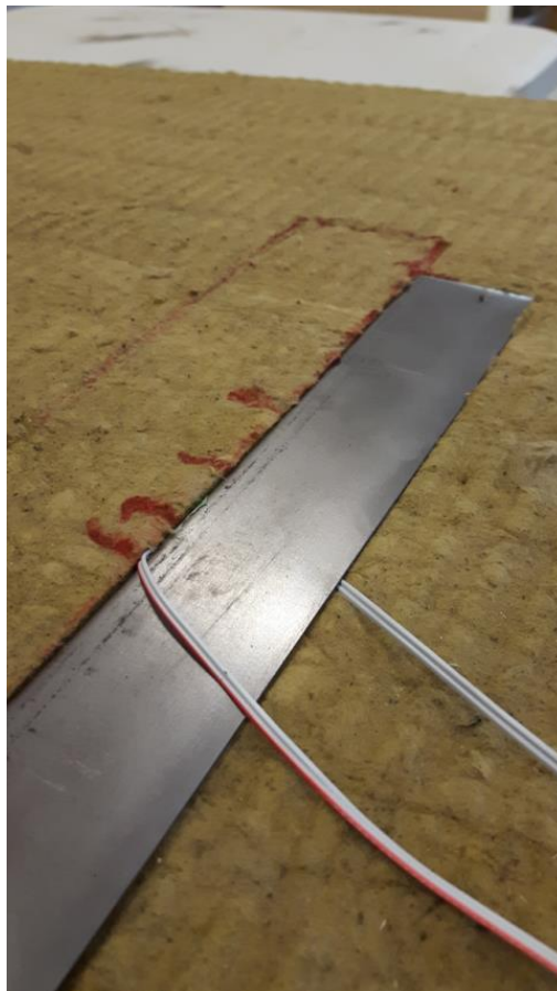
Detailed view of the Z-girt in the insulation.
