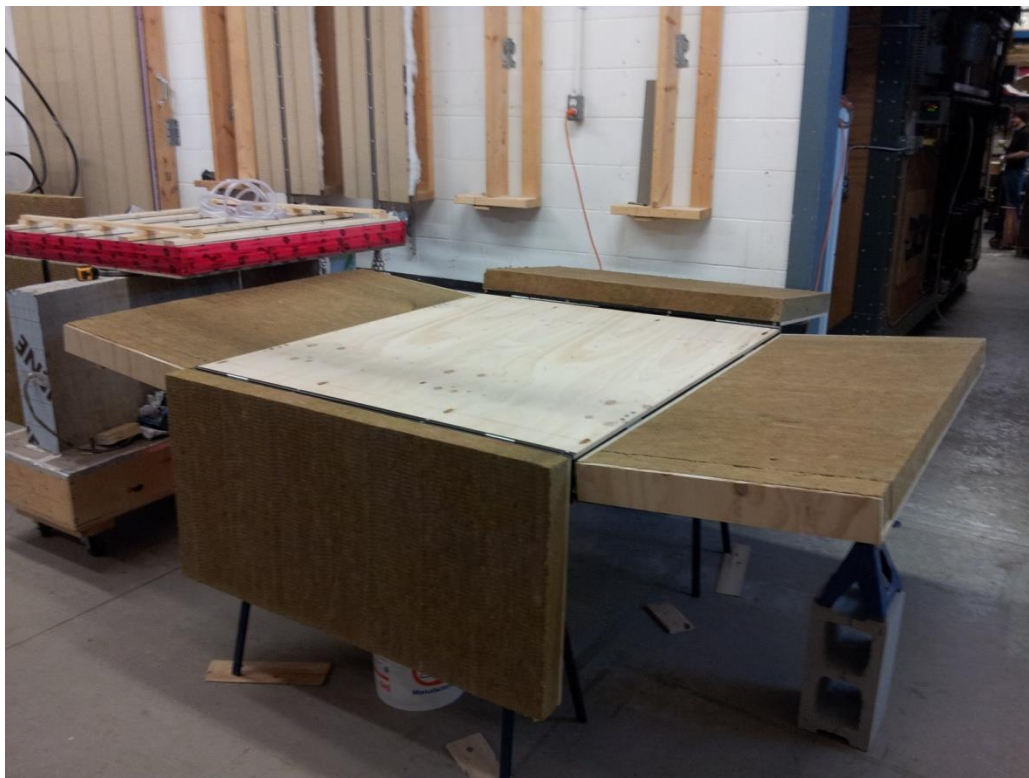
Edge insulation installed.
