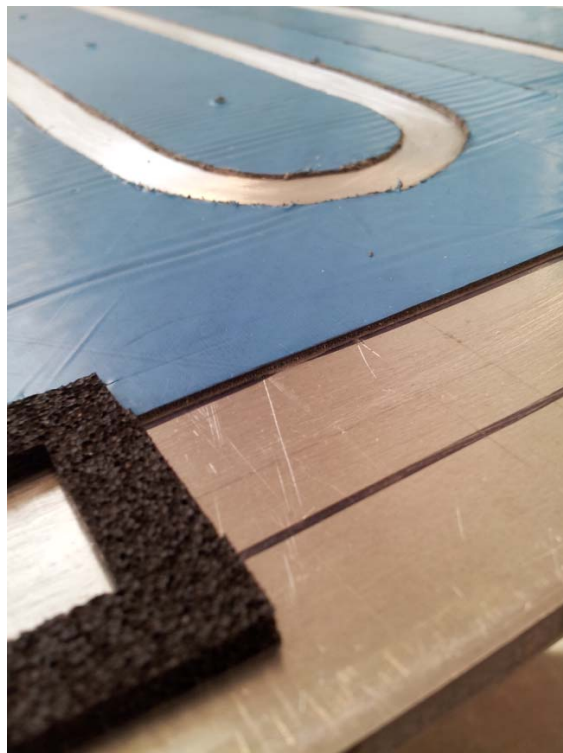
Figure 19 – A detailed view of the Blueskin WP® used to act as formwork for the epoxy.
