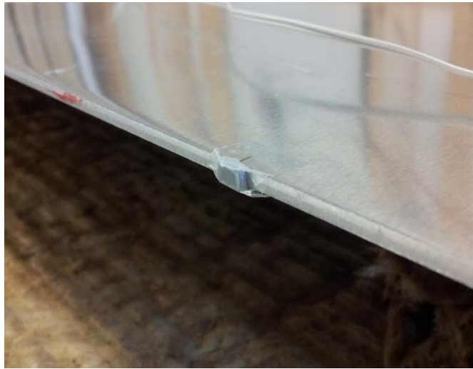
Figure 9 – Guard gap spacers.
