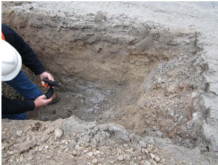
Figure 3-3: View of excavated test pit showing shale subgrade material
