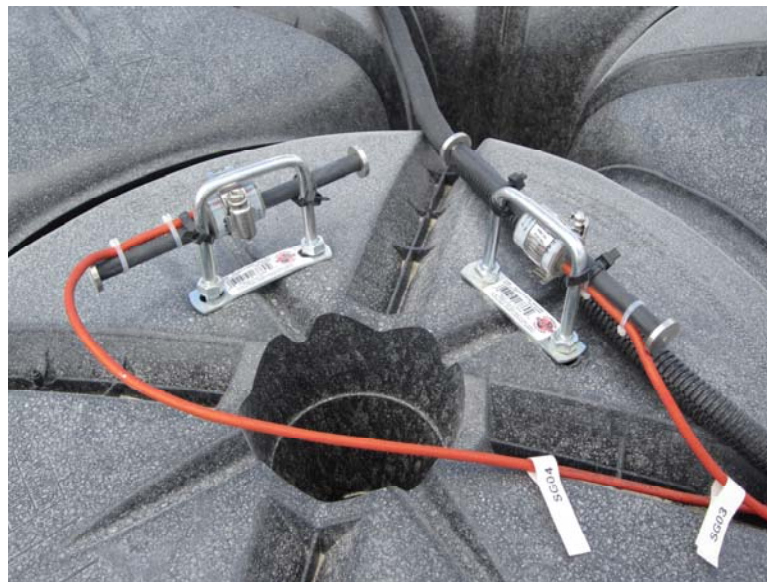
Figure 3-10: Arrangement of strain gauges on Cupolex® unit
