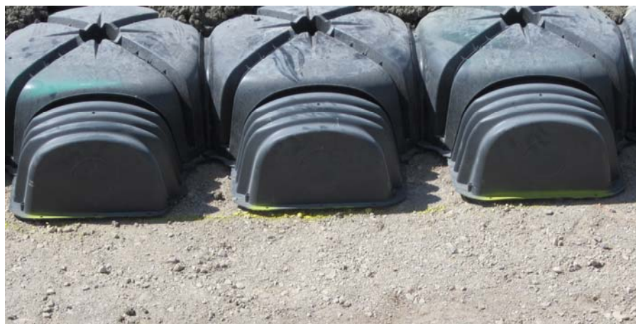
Figure 3-7: Installed BetonStop® products, doubled up to prevent punchout
