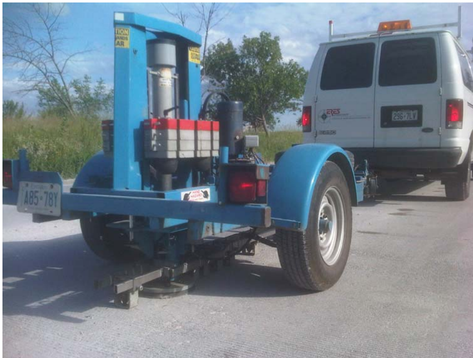
Figure 4-11: Falling Weight Deflectometer testing in progress
