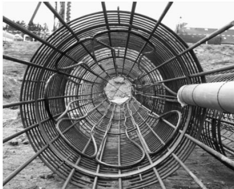
Figure 1-3 Pile reinforcement with absorber pipes (Brandl, 2006)
