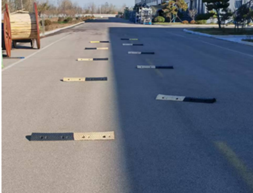
Figure 4.21: Multiple Sets of Cross Speed Bumps
