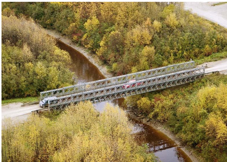
Figure 2-1: Bailey Bridge Spanning Buttler Creek, Moosonee [Paul Lantz 2006]
