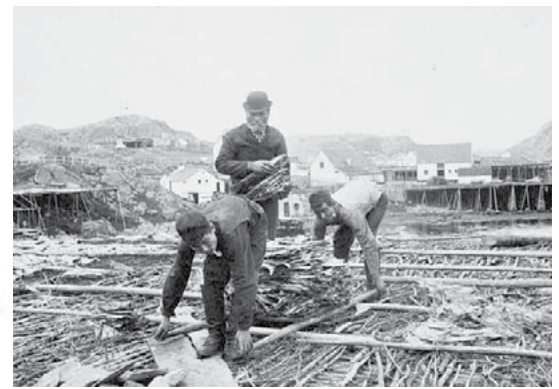
Fig. 3.5 Drying and salting cod in the early fishery, 1886. Called flakes, these structures of logs and sticks were designed for air drying the fish.
