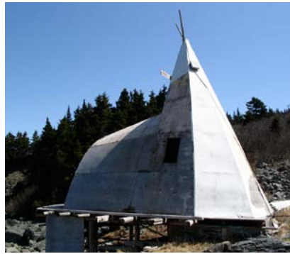
Fig. 3.33 Marine technologies, such as fibreglas on wood show promise for maintaining the properties of light, flexible wooden architecture.
