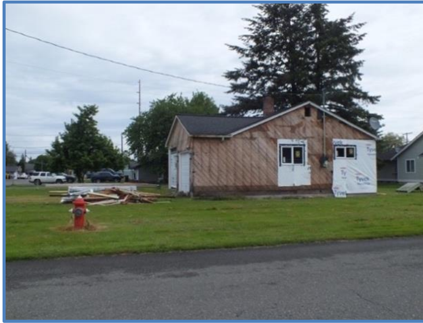
Figure 24: Home repairs were ongoing in Sumas, WA over 1 year post-AR (Watterodt, June 2022)
