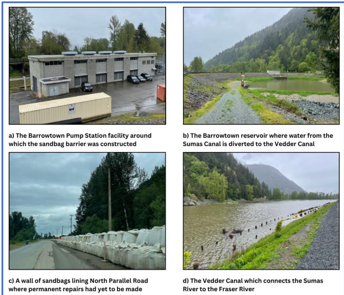
Figure 18: Barrowtown Pump Station and the Vedder Canal (Watterodt, May & June, 2022)
