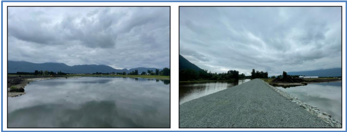
Figure 22: Flooded farmland at dike breach site (Watterodt, June 2022)
