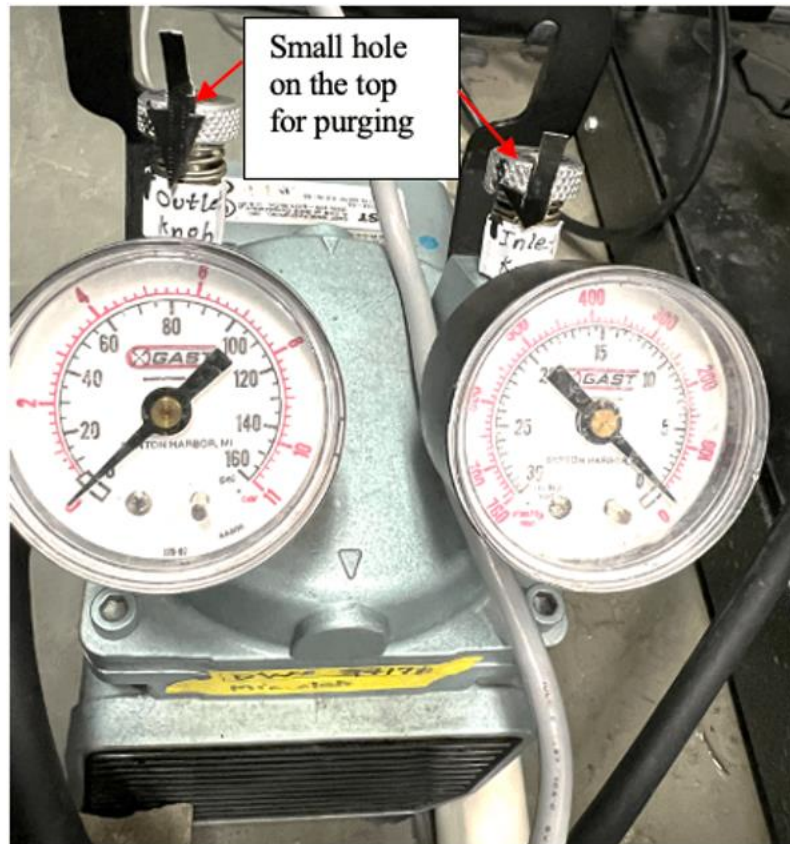
Figure A.7 Image showing the markings on the air compressor
