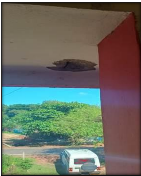
Figure 6: Gabakund Cyclone shelter (Top), Presence of cracks in the shelter roofs (Down, left), and Condition of Washbasin and Washroom (Down, right) (Photo: Greeshma Prakash Sherly).
