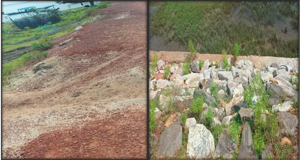
Figure 4: The condition of barriers in Parbatipur (eroded and not in sufficient height) (Left) and the images of proper barrier walls in Mirjapur (in the same extend) (Right) (Photo: Greeshma Prakash Sherly)
