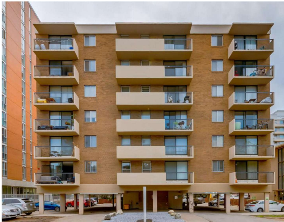
Figure 3.3: The 1970s Case Study Mid-Rise Multi-Unit Residential Building
