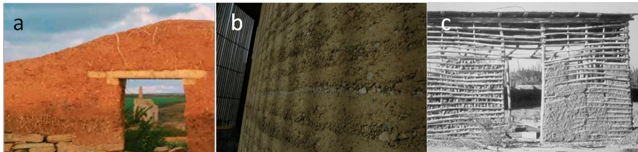
Figure 1: Traditional construction techniques using earth a) A cob wall constructed in Mount Pleasant Eco-Park, Cornwall (United Kingdom) 2 b) Unstabilized loadbearing rammed earth (Berlin) 3 c) Wattle and Daub building (Venezuela) 4
