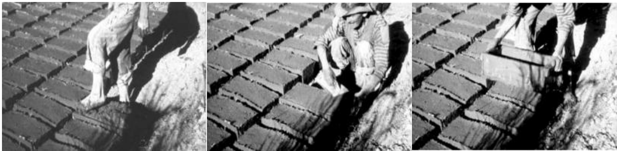
Figure 2: Adobe bricks being made and left to dry (Ecuador) 4
