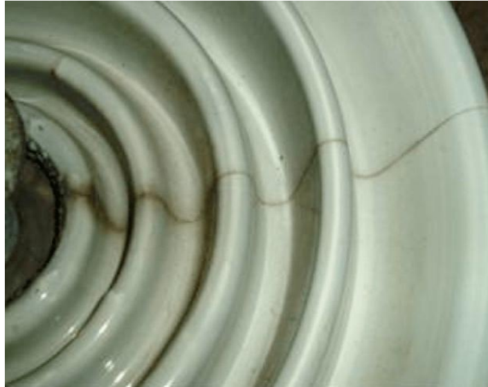
Figure 1.5 A radial crack in a ceramic insulator sample due to Portland cement expansion [12]
