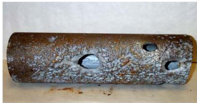
Figure 2.1 - Material degradation (pipe corrosion) (Adapted from Knight , 2013)
