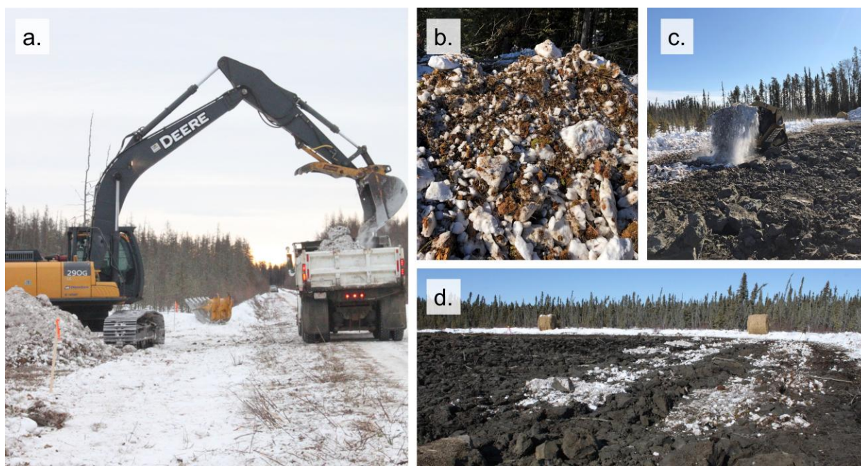
Figure A.2: Photos of the vegetation propagule collection process (a), vegetation propagules prior to introduction onto the site (b), spreading of the vegetation propagules using a skid-steer (c), and propagules introduced directly onto the roughened residual mineral substrate (d). All photos were provided by the Northern Alberta Institute of Technology (Centre for Boreal Research).
