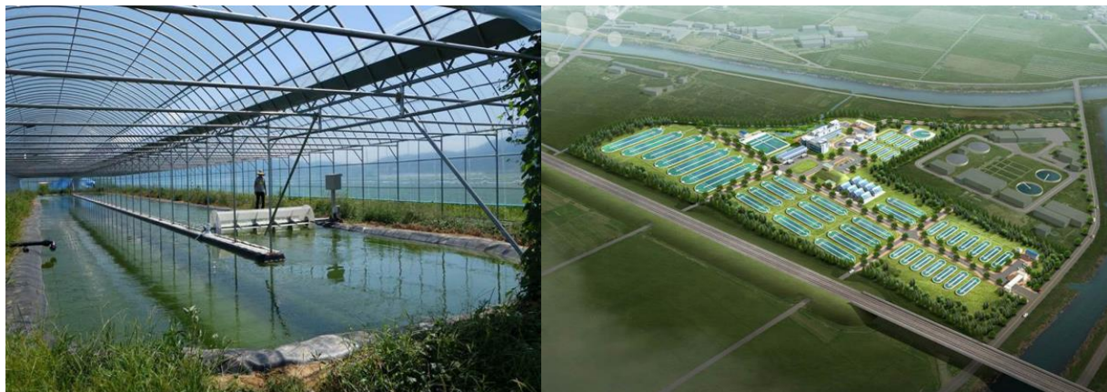
Figure 8 a) Experimental raceway pond in a glass greenhouse at Chilgok-gun Agricultural Technology Center (Yoon, 2012), b) Design drawing of the algae biofuel pilot plant (Gyeongsangbuk-do, 2010)
