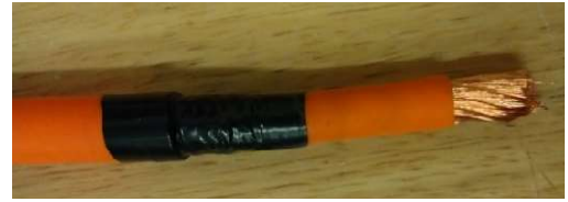
Figure 12: HV cable ready for crimping with shielding and outer insulation stripped further back and taped
